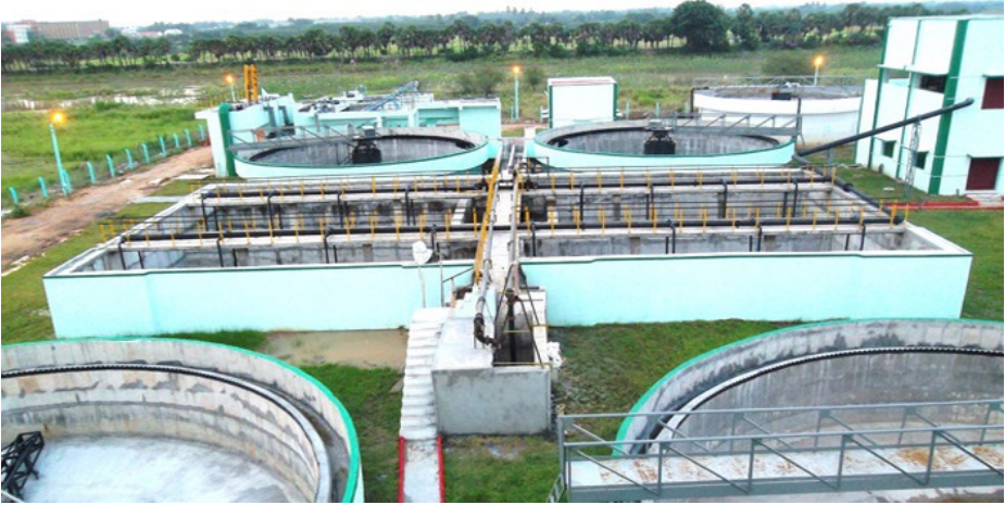
WWTP at Chennai 1
